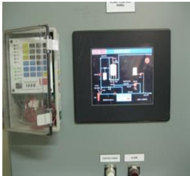
Figure 4-4a Ion Exchange Treatment Equipment (single exchange vessel)
