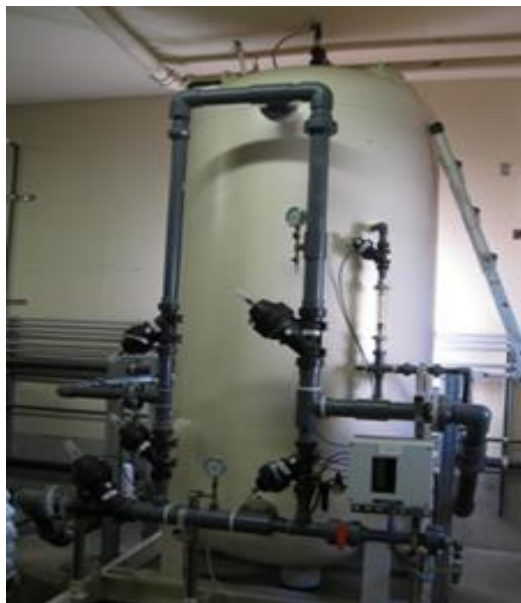
Figure 4-4a Ion Exchange Treatment Equipment (single exchange vessel)
